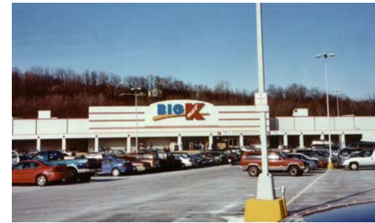
Big Kmart at Mark Plaza, Edwardsville
